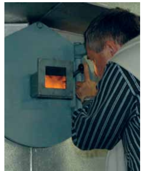
Anatoly Lukin from Archangel inspects a heating plant in Mynämäki.
