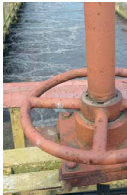
The project in Sosnovy Bor will reduce the discharges of phosphorus by some 22 tonnes per year.
